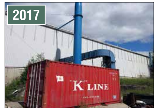
GREENHECK Paint Area 50 hp Dust Collector
